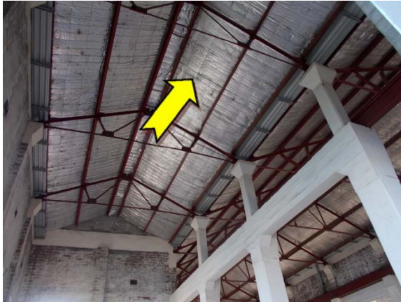
Photo 1. Interior, throughout, roof, insulation – suspected SMF sarking insulation material.
